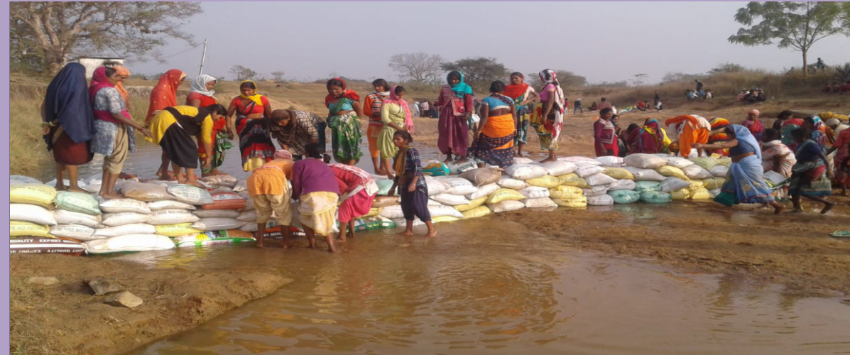
Women making Temporary dam under DFW
